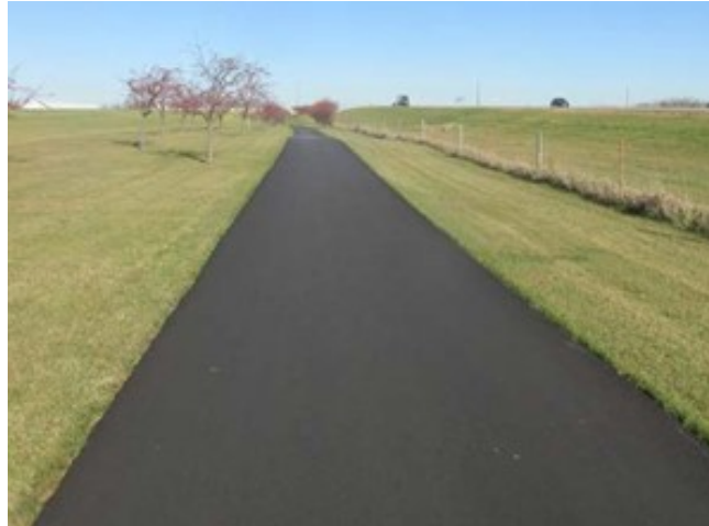
Figure 12-5: An asphalt overlay on top of an existing asphalt path, which previously had a deteriorated
